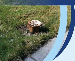
Effects of a harsh winter may be noticed in the landscape long after the snow is gone. Frost heaving sometimes lifts natural gas and water standpipes out of the ground, creating a potential safety hazard.
