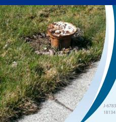
Effects of a harsh winter may be noticed in the landscape long after the snow is gone. Frost heaving sometimes lifts natural gas and water standpipes out of the ground, creating a potential safety hazard.
