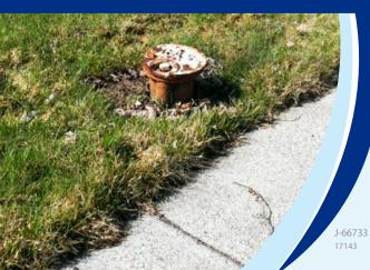
Effects of a harsh winter may be noticed in the landscape long after the snow is gone. Frost heaving sometimes lifts natural gas and water standpipes out of the ground, creating a potential safety hazard.
